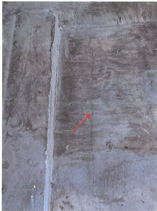
Photograph No. 38 - Fissure in the reinforced concrete beam near its support.
