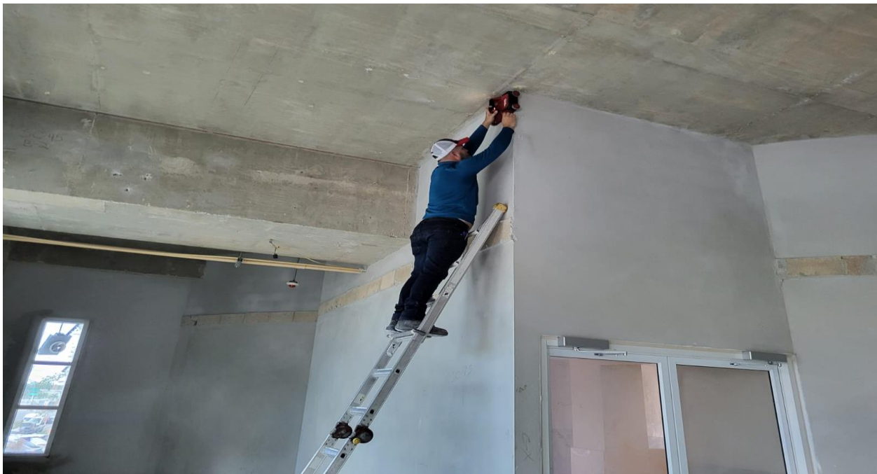
Photo 4: Performing scanning on CMU walls.
