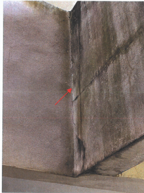
Photograph No. 12- Fissures along the connection between the reinforced concrete parapet and the parking building reinforced concrete parapet
