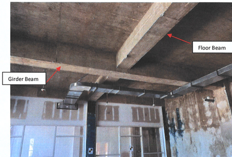
Photograph No. 5 -Typical reinforced concrete girder supporting reinforced concrete beam, Axis 5' between Axis F and Axis H
