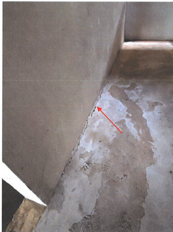
Photograph No. 10 – Fissures were found along the construction joint, at Axis 8, in every level
