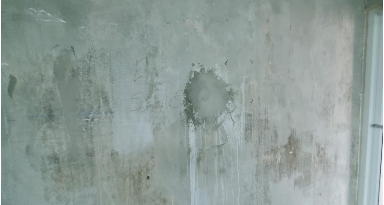
Photo 13: After core extraction, holes were backfilled with high strength structural mortar.
