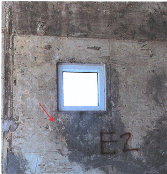
Photograph No. 13 – Fissures radiating from the corners of the window opening located in the Shear Wall
