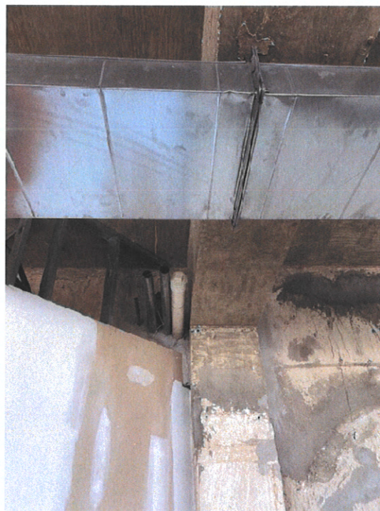
Photograph No. 30- Concentration of pipes and conduits at a reinforced concrete beam between the shear walls Axis F. The ACI 318 building code requires a minimum spacing between pipes or conduits at 3 times the diameter of the pipe
