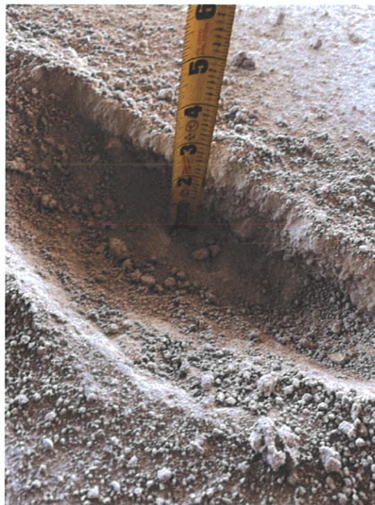
Photograph No. 28 – A hole was found in the slab topping, approximately 2-1/2" of topping was used to level floors in that area, could be more
