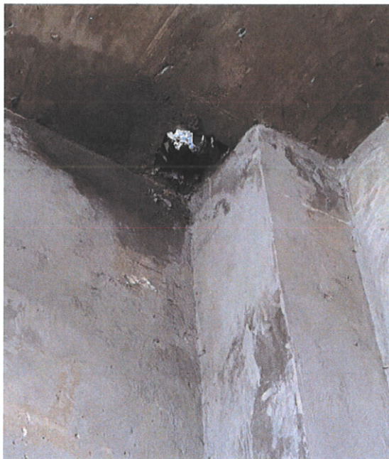
Photograph No. 20 - Opening through the reinforced concrete slab
