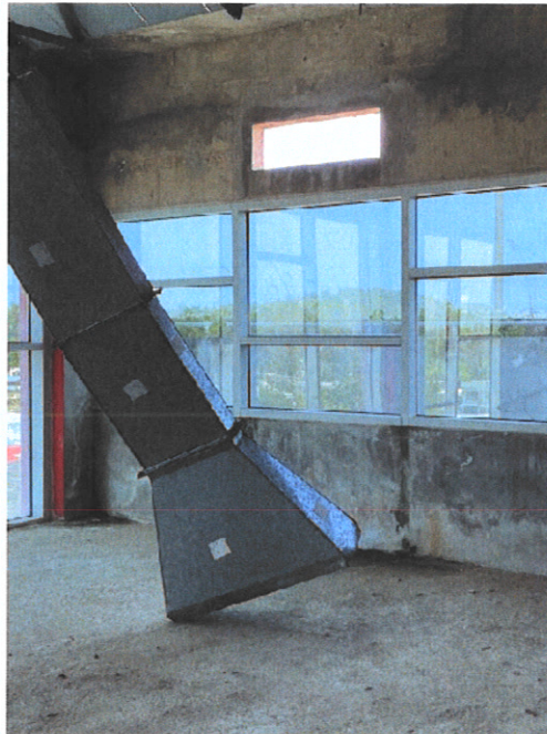
Photograph No. 34 – This opening for the A/C ducts in this beam occurs in every level , at Axis 7, between Axis G and Axis H. The strucutral drawings indicated a shear wall in this Axis
