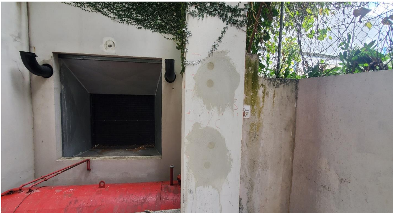
Photo 14: After core extraction, holes were backfilled with high strength structural mortar.
