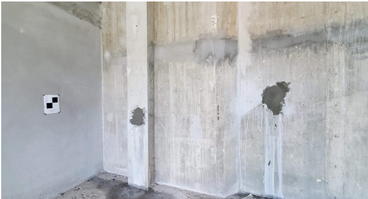
Photo 12: After core extraction, holes were backfilled with high strength structural mortar.
