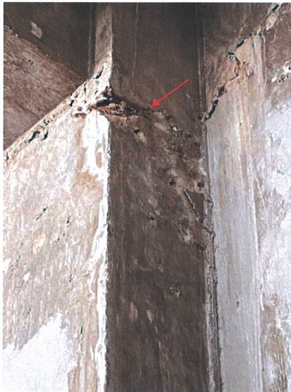
Photograph No. 8 – Construction joint showing debris between concrete pours
