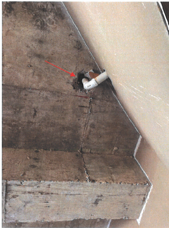
Photograph No. 35 – Drainage pipe at roof level, opening in the slab was poorly done after slab was already poured
