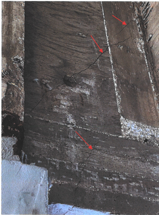
Photograph No. 29 – A closeup of picture 16 illustrating the fissures in the spandrel beam that support the girder beams, near its support to the column.
