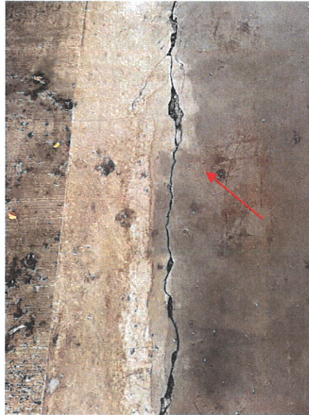
Photograph No. 9 – Fissure along Axis 8 where there is supposedly a construction joint.
