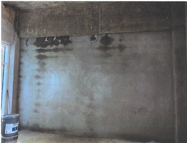
Photograph No. 25 – This exterior cement block partition wall was shown in the structural drawings as a reinforced concrete shear wall
