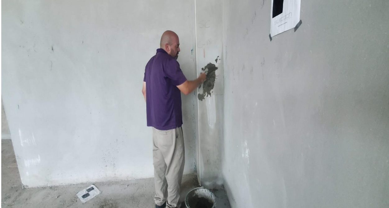
Photo 11: After core extraction, holes were backfilled with high strength structural mortar.
