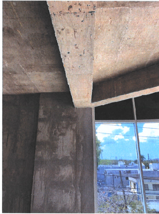
Photograph No. 17- Repaired reinforced concrete column
