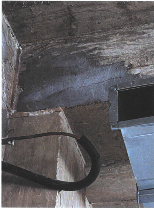
Photograph No. 31 - Mortar placed to cover some deficiency in the existing reinforced concrete beam, this occurs at the Fourth Level, Axis D -3
