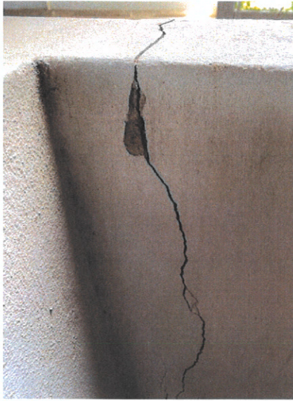
Photograph No. 33 – Crack in parapet beam in exterior stairs area, where the construction joint is located
