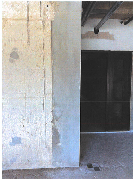
Photograph No. 26 – This reinforced concrete column was repaired?? Most likely it was not poured properly when concrete was placed, creating voids in the structural member
